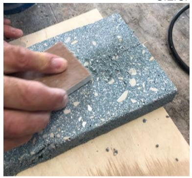
3. Remove any larger deposits of material from the surface but leave the material slightly proud over the surface of the crack.
