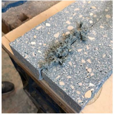
2. Using the piece of SilicaStone supplied with the repair dust, rub the resin in a circular motion forcing the material into the crack, you should continue to do this until as much of the material has been forced into the crack as possible.
